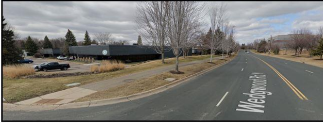
Maple Grove office / warehouse 01
