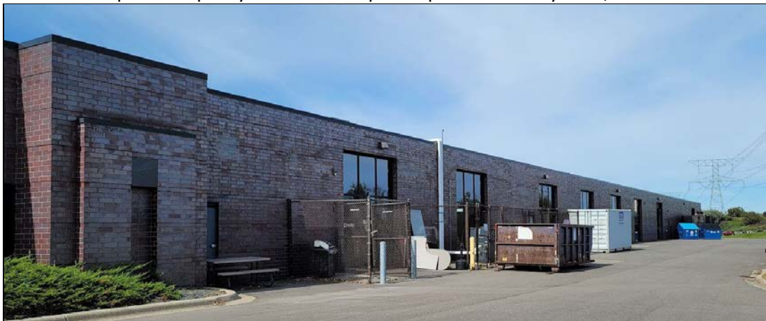
BACKSIDE OF MAPLE GROVE WAREHOUSE
