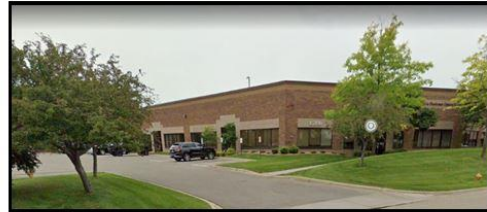
Plymouth office / warehouse 01
