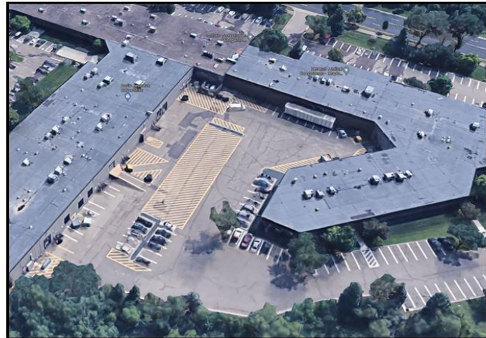
Maple Grove office / warehouse 02 overhead / back
