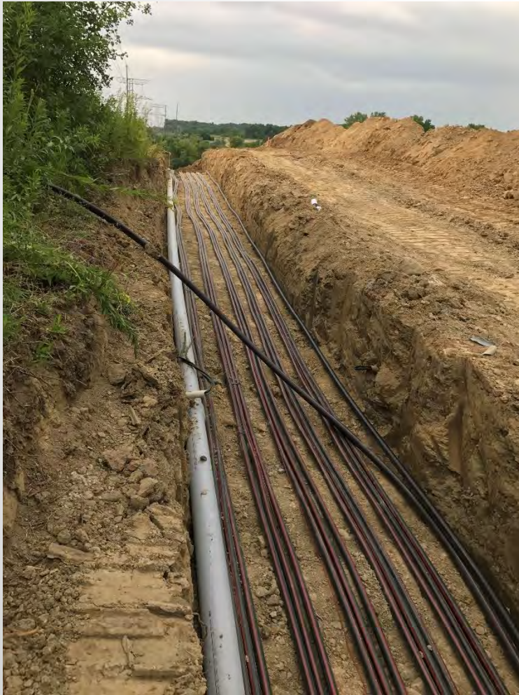
Future installation along Co Rd 116
