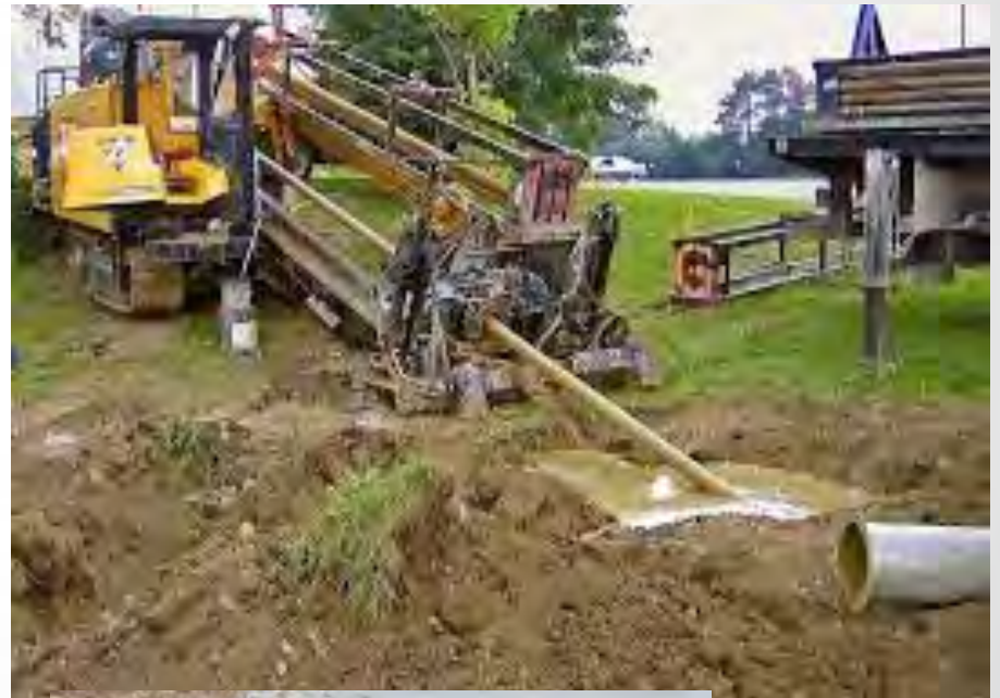
installation along Larkin Ave
