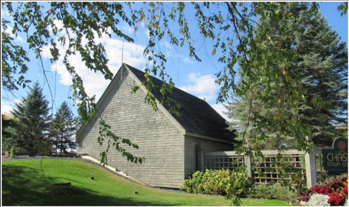
Chaska Ground Water Storage Booster Station
