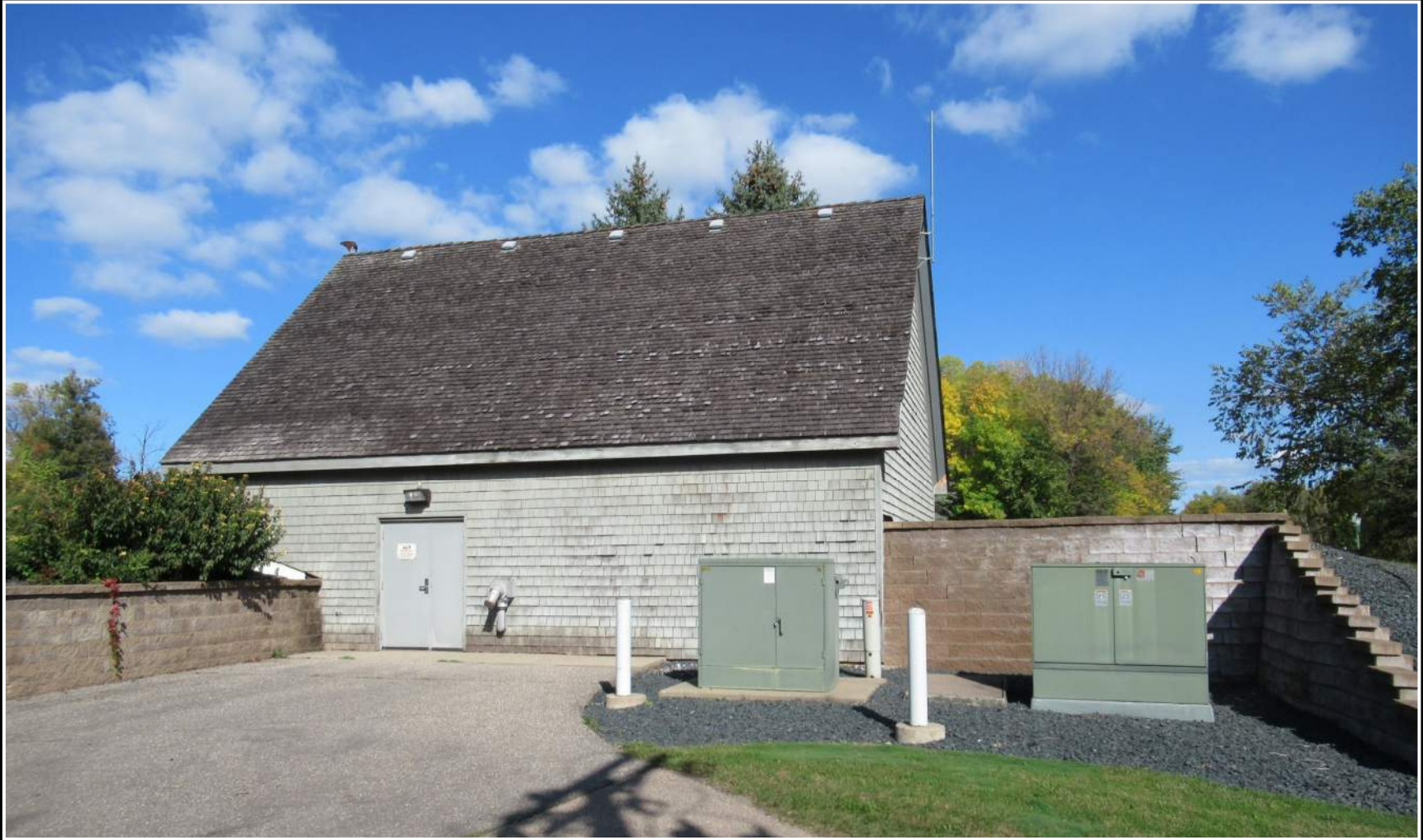
Chaska Ground Water Storage Booster Station
