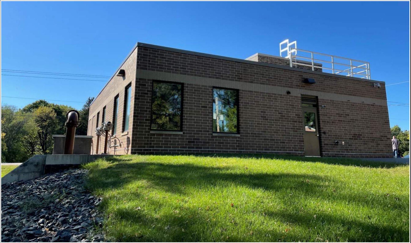
Stacy Water Treatment Facility
