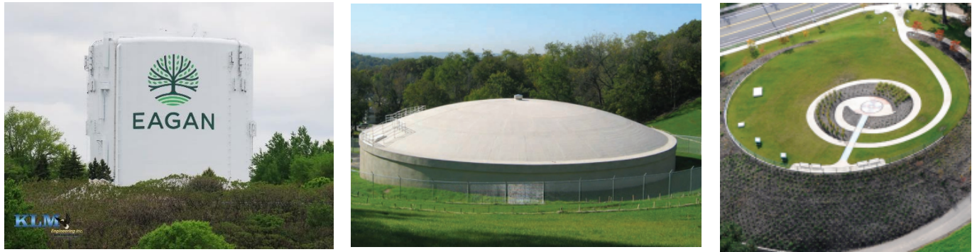
Figure 3: Ground Storage Tank Examples
