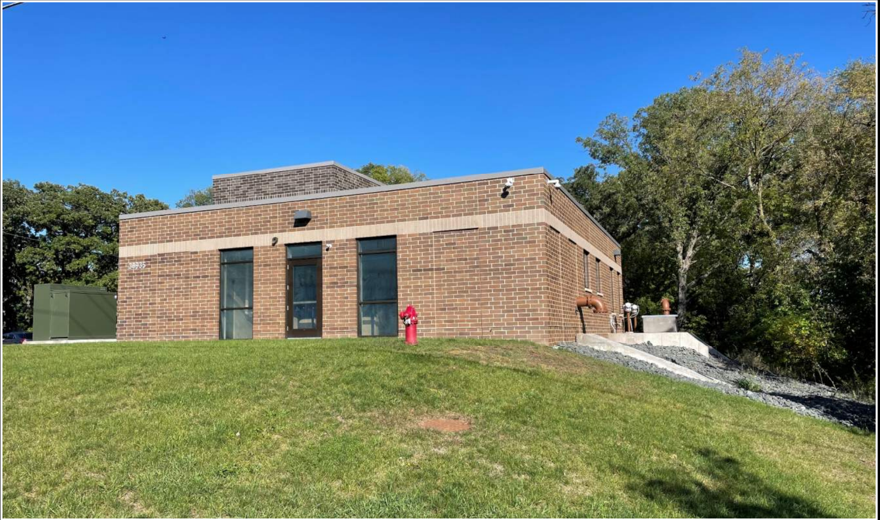
Stacy Water Treatment Facility
