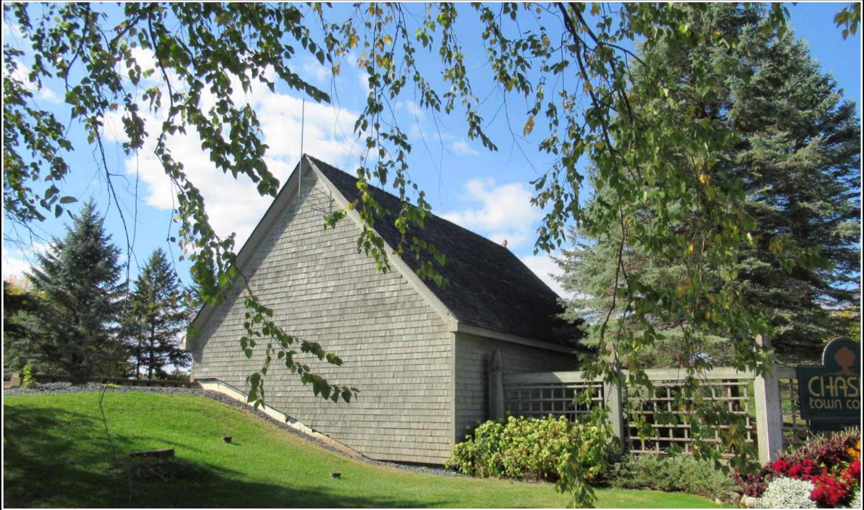
Chaska Ground Water Storage Booster Station
