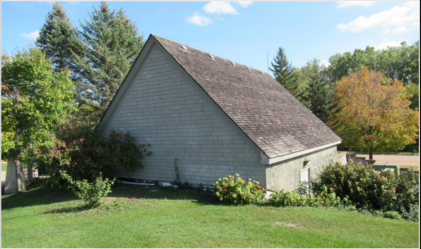
Chaska Ground Water Storage Booster Station
