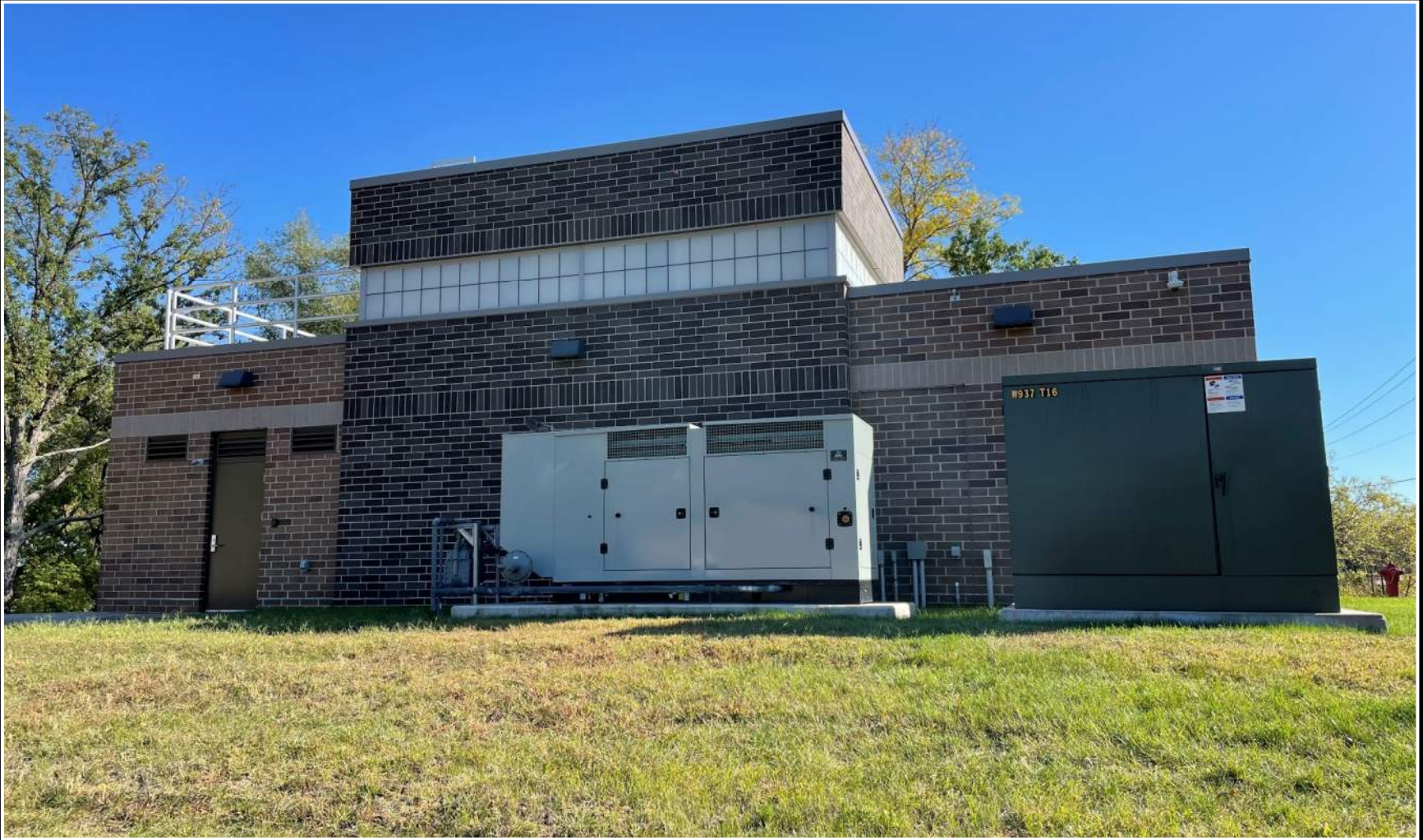
Stacy Water Treatment Facility
