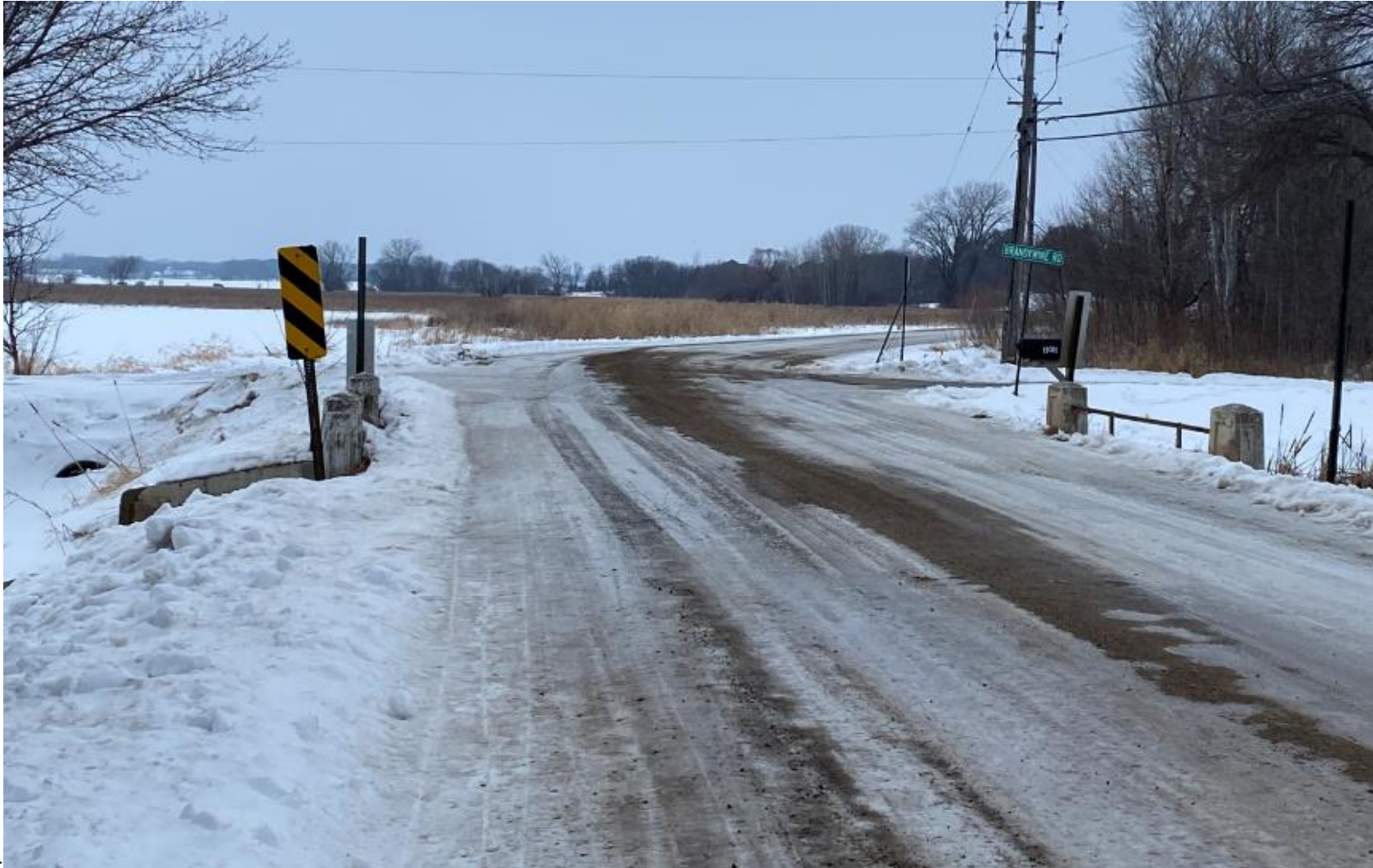
Schutte Road - Looking West
