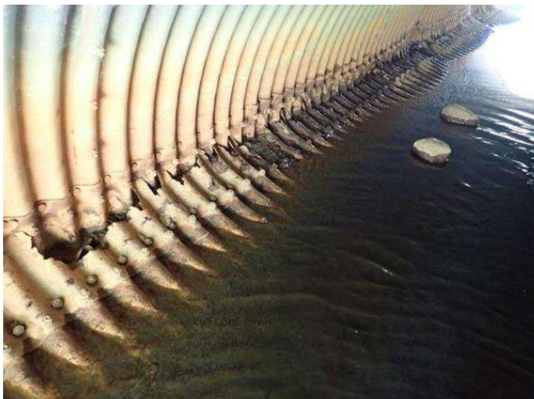
Trail Haven Road – Loss of Section
