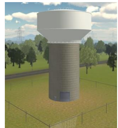
Figure 5-2 Composite Water Tower (courtesy of KLM Engineering)
