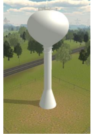
Figure 5-3 Single Pedestal Water Tower (courtesy of KLM Engineering)
