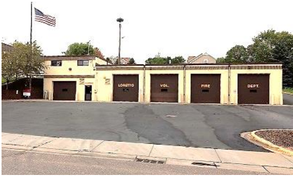
Figure 15: Loretto Fire Station
