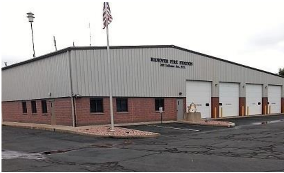
Figure 14: Hanover Fire Station
